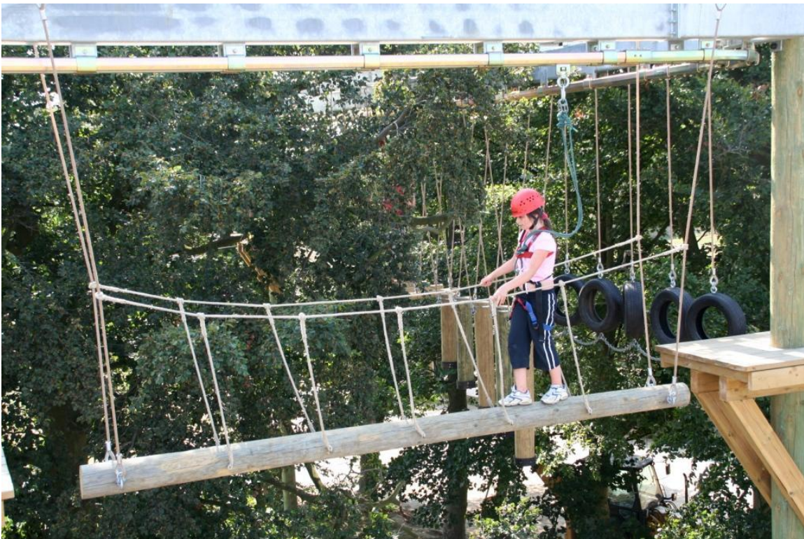
Continuous Belay (rail system)
